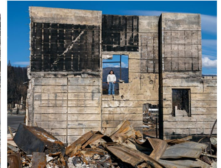
Danielle Guerra at the site of the Sierra Lodge Hotel in downtown Greenville, where she had worked and lived. She and her sister made a narrow escape as the flames tore through the town destroying around 80% of the structures. Taken on 31 October 2021.
